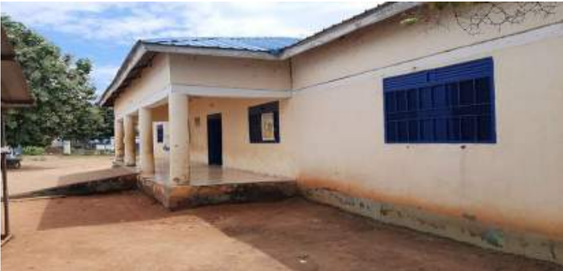
New Site center before renovation
