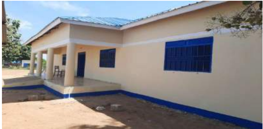
New Site center after renovation
